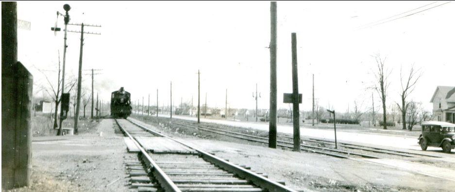
Woodward at 12 Mile Looking South—March 1930
